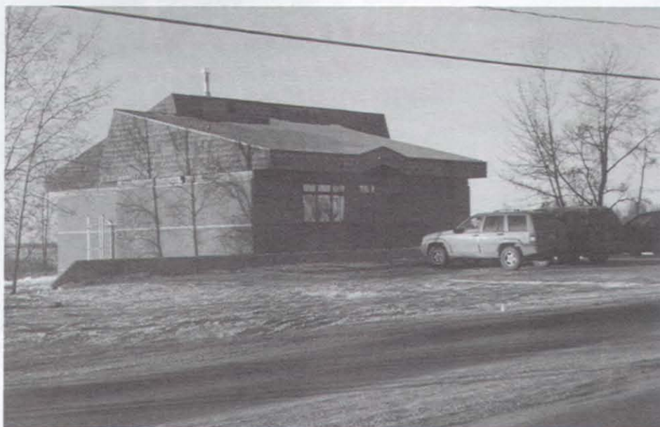
La Loche Village Office
